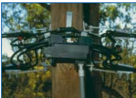
Opening a switch using hook stick
