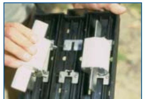
Replacing a fuse link
