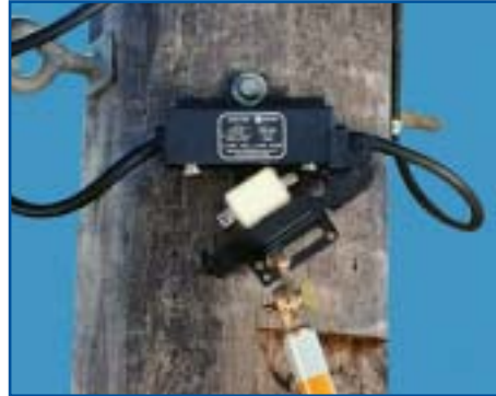
Hook stick operation on single pole version
