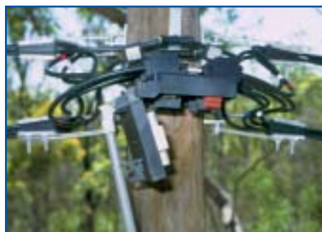
Removing lower housing using hook stick
