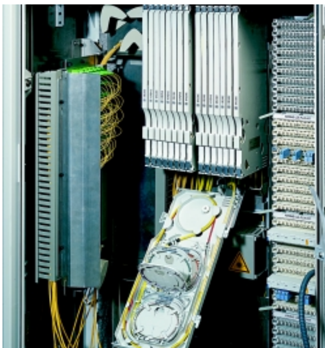
Pict 1: Patch field swivelled open and open tray housing with FAME6
